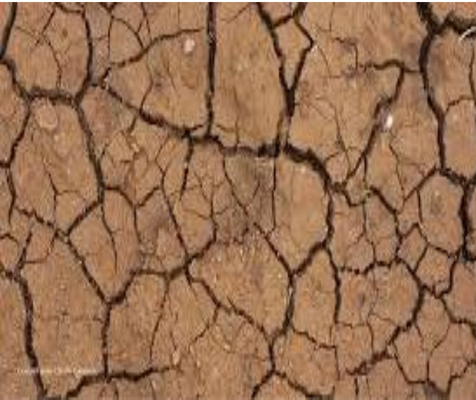
Cracking of soil
