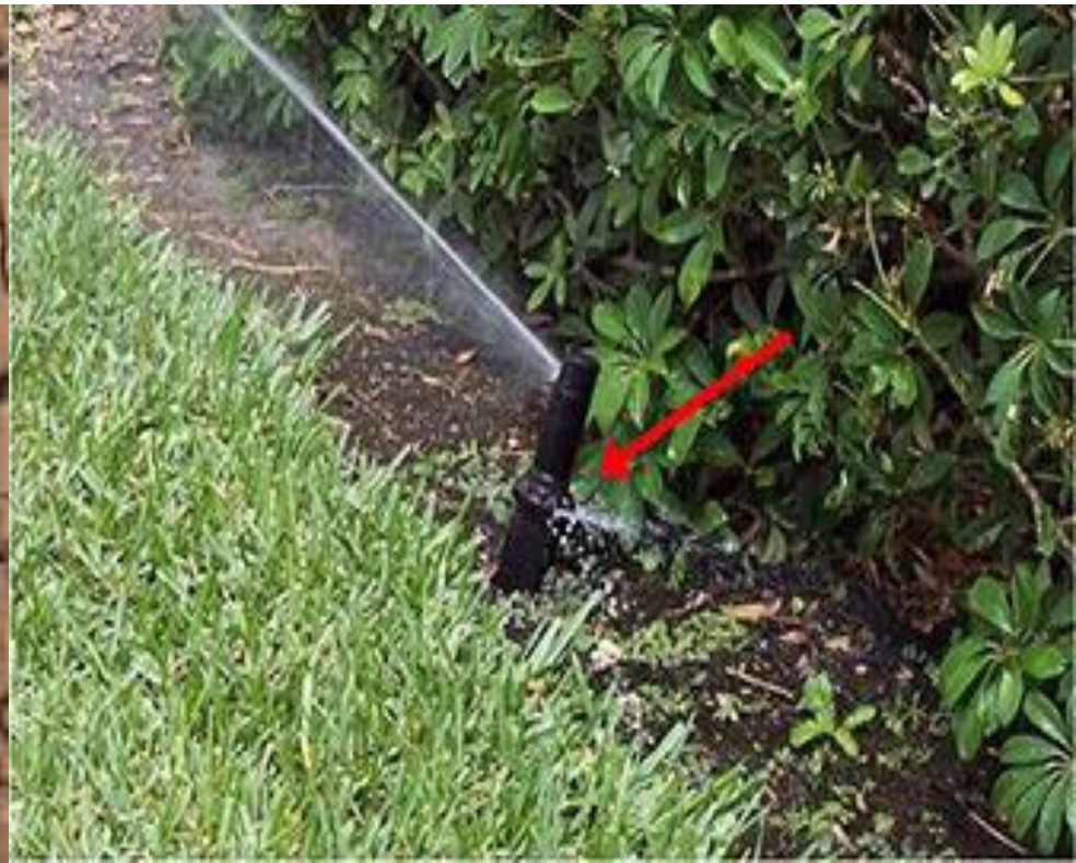
Leaking Sprinklers
